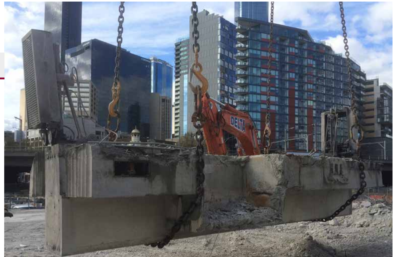
ABOVE - Winged structural beam removal.
